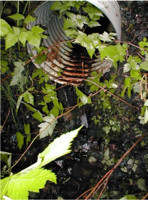
Figure 13. A remediated red pipe at 3015000 MP 0.344. Before photo (left) shows a 36 inch pipe that is perched and is installed at a steep gradient. After photo (right) shows a 96 inch pipe that has had bedload placed inside the pipe simulating a stream bottom.
