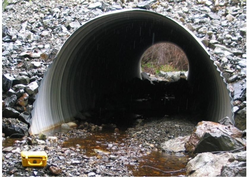
Figure 13. A remediated red pipe at 3015000 MP 0.344. Before photo (left) shows a 36 inch pipe that is perched and is installed at a steep gradient. After photo (right) shows a 96 inch pipe that has had bedload placed inside the pipe simulating a stream bottom.
