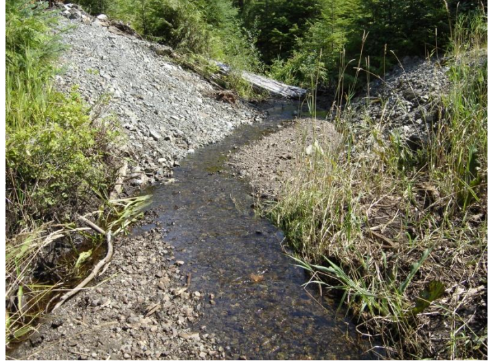
Figure 14. A red pipe removed at 3015105_0.96L MP 0.038. Before photo (left) shows 36 in pipe that is crushed and buried in the road prism. After photo (right) shows downstream view of removed crossing due to proper road storage.
