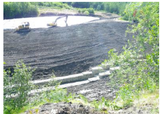
RDM after interim stabilization efforts were completed to reduce mobilization of mine tailings into the creek.
