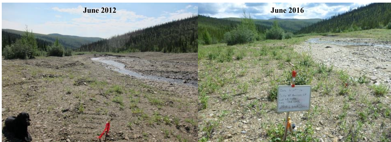
Reclamation completed in 2010 is still lacking lateral stability, bedform diversity, and riparian vegetation.
