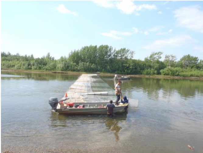
Floating resistance board weir on the Unalakleet River provides critical information to BLM Alaska regarding salmon escapement.
