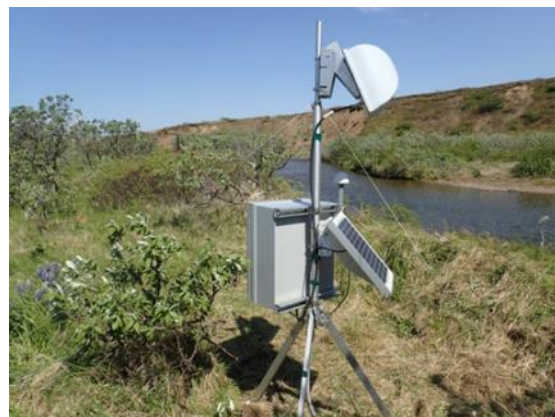
Satellite transmitter at Platinum Creek.
