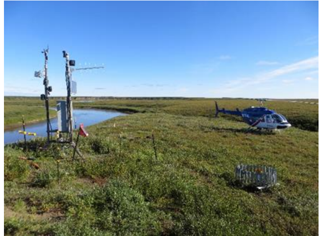
Stream gage site within the NPR-A.
