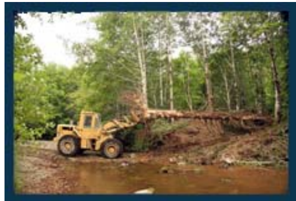
Figure 17. Moving large woody debris into the stream channel to re-establish structure in a 1-mile stretch of Sal Creek
