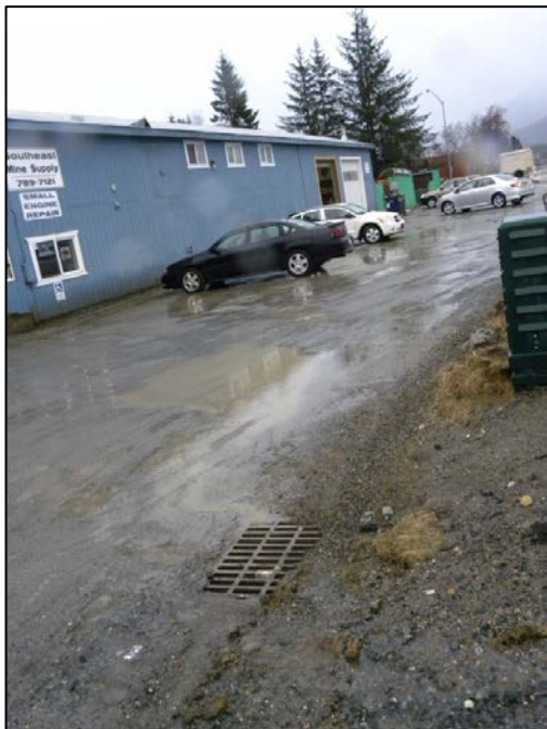
Figure 23. Turbid stormwater from a gravel parking area flows into a catch basin at the intersection of Crest Street and Airport Blvd.
