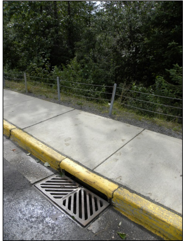
Figure 5. Curb and gutter systems are commonly used to direct runoff from roads and parking lots into catch basins.
