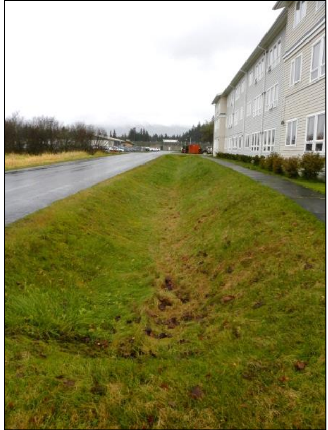
Figure 7. A swale at the south end of Alpine Avenue.
