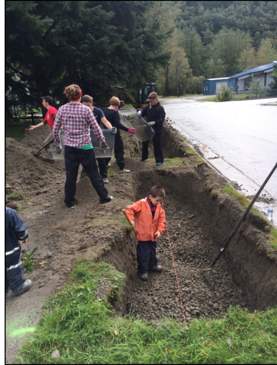
Figure 31. Infiltration basins under construction near Pullen Creek in Skagway. Curb cut-outs intercept runoff in the gutter allowing stormwater to flow into the basins rather than flowing directly into Pullen Creek.
