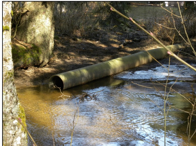
Figure 13. North Jordan Avenue Outfall #3.
