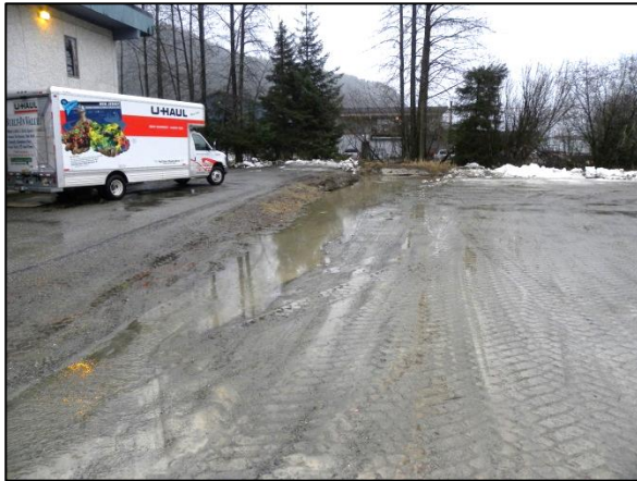
Figure 15. Stormwater runoff from a portion of the Airport Shopping Center parking lot flows over an unpaved area used to train truck drivers next to Jordan Creek. (view looking east).
