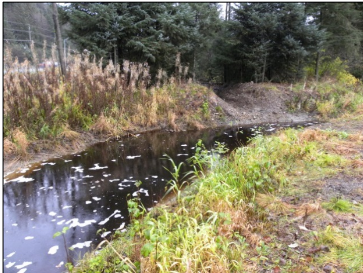
Figure 8. An infiltration basin at the north end of Jordan Avenue during a runoff event.
