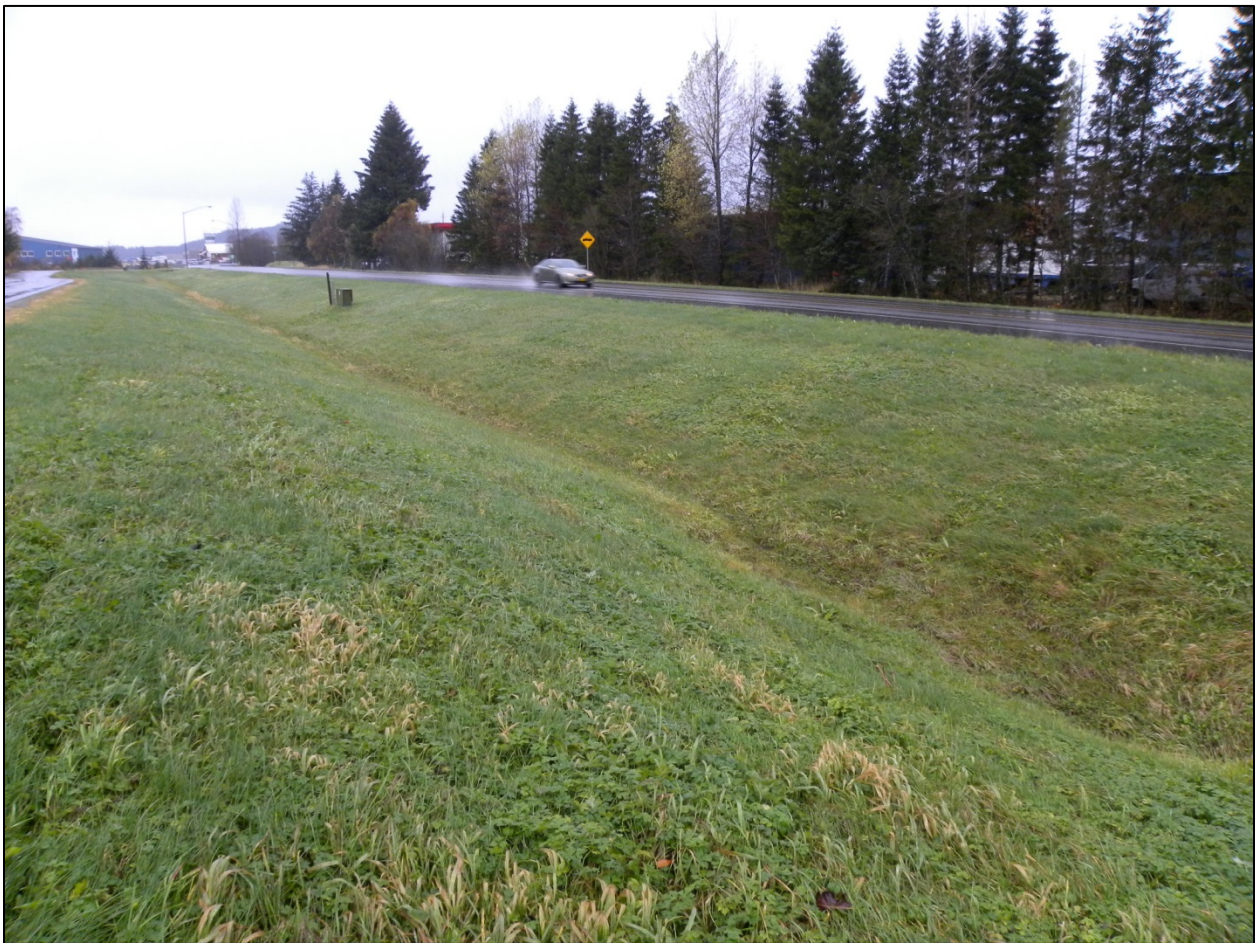
Figure 24. A 1,500 foot long swale at the east end of Yankukin Drive. If feasible, stormwater from the Crest Street stormwater system - the largest system in the assessment area - could be routed to this swale instead of flowing directly into Jordan Creek.
