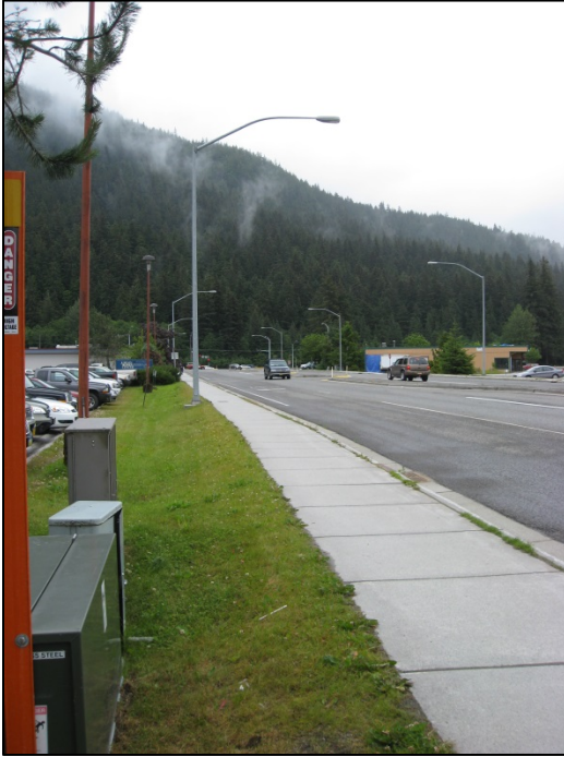
Figure 30. Route curb and gutter stormwater away from catch basins and into filtration strips constructed in green spaces next to roads (view looking east along Glacier Hwy. near Jordan Avenue).
