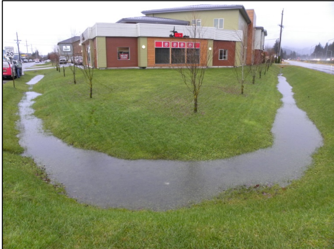
Figure 26. Grass-covered swales at the intersection of Airport Boulevard (left) and Old Dairy Road (right) promote infiltration of stormwater runoff when the ground is unfrozen.
