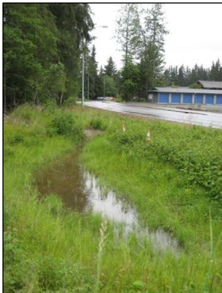
Figure 10. An infiltration basin located near the north end of Jordan Ave receives stormwater runoff from roof tops and asphalt surfaces (view looking south).
