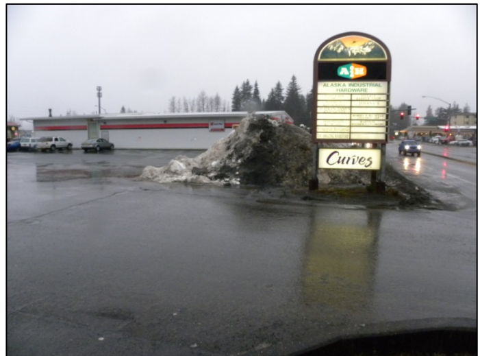
Figure 29. Suspended sediment from a snow pile is carried by meltwater runoff into catch basins within the West Glacier Highway stormwater system.
