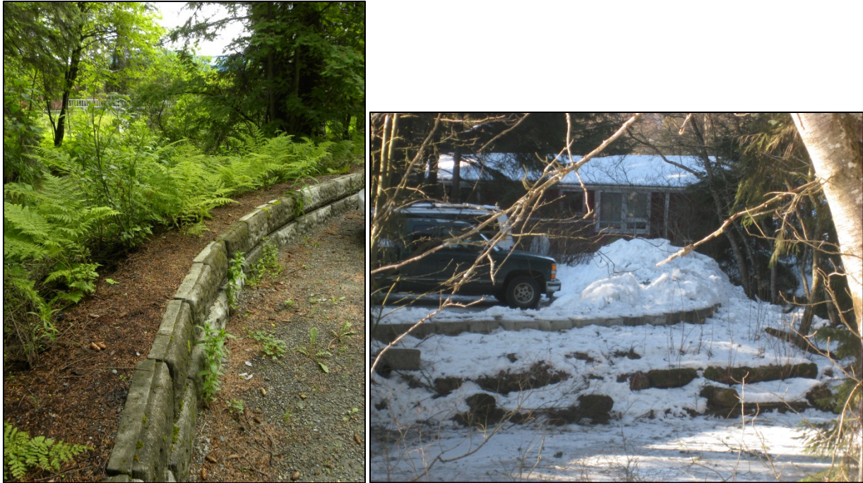
Figure 28. A snow barrier constructed of precast concrete blocks prevents snow from being plowed onto riparian habitat at a business parking area next to Jordan Creek.
