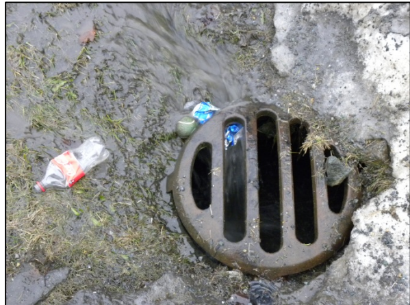
Figure 22. Stormwater flows into a catch basin in the northeast corner of the Nugget Mall parking lot.
