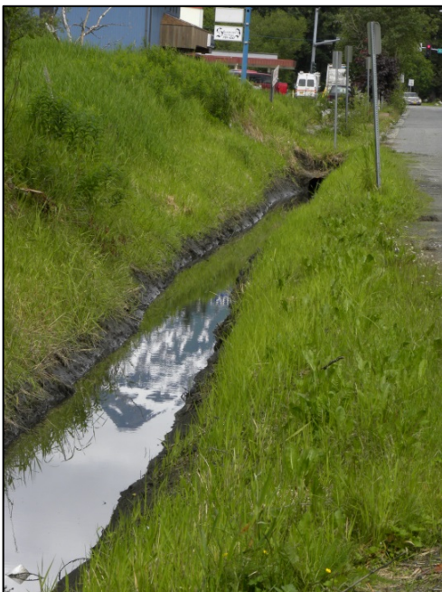
Figure 32. Ditch cleaning removes vegetation that prevents soil erosion and promotes sedimentation (view looking north from the south end of Jordan Avenue).
