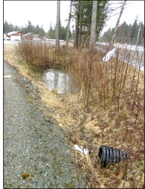
Figure 9. An infiltration basin near the north end of Jordan Avenue. The outlet pipe ( lower right) connects the basin to a ditch along Egan Drive.
