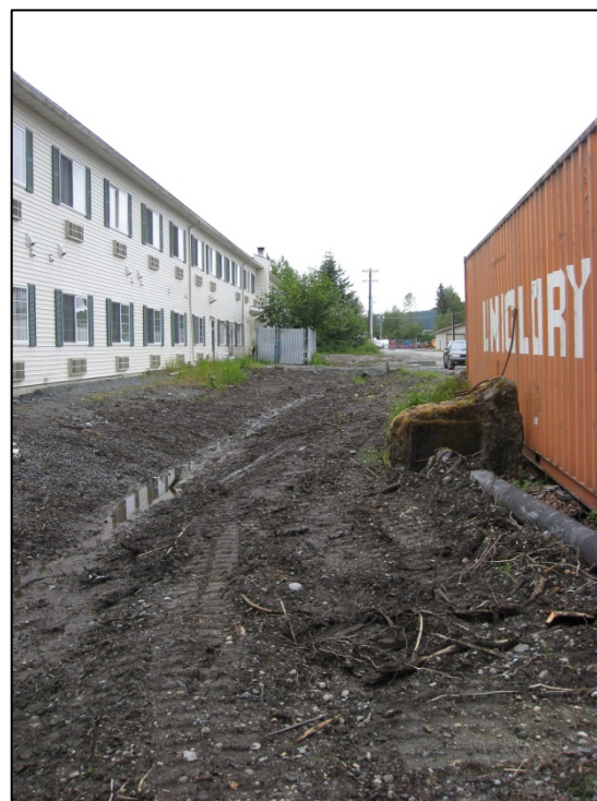
Figure 17. This shallow ditch on the north side of the Extended Stay Hotel is underlain by a french drain (view looking west).
