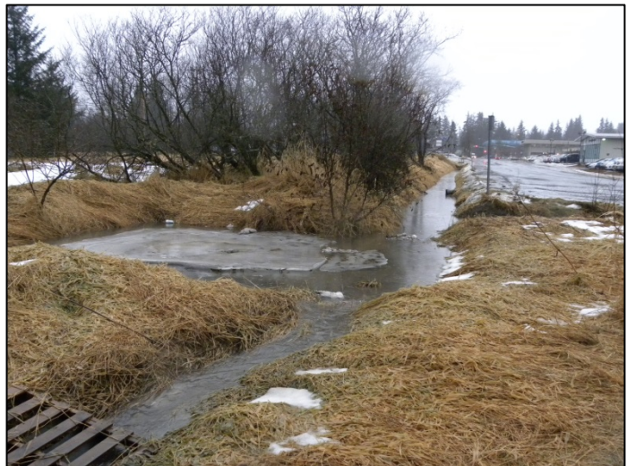
Figure 19. The Nugget Mall South stormwater ditch conveys stormwater from the south side of the mall into a small retention basin (center left in photo) before it flows into Jordan Creek at the south end of Jordan Avenue (view looking north from Jordan Creek).
