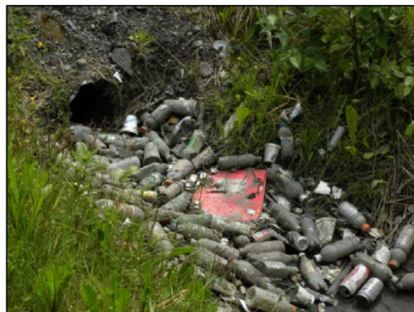
Figure 12. Litter from the Trout Street ditch accumulates at a culvert outfall (Outfall 3) next to Jordan Creek.
