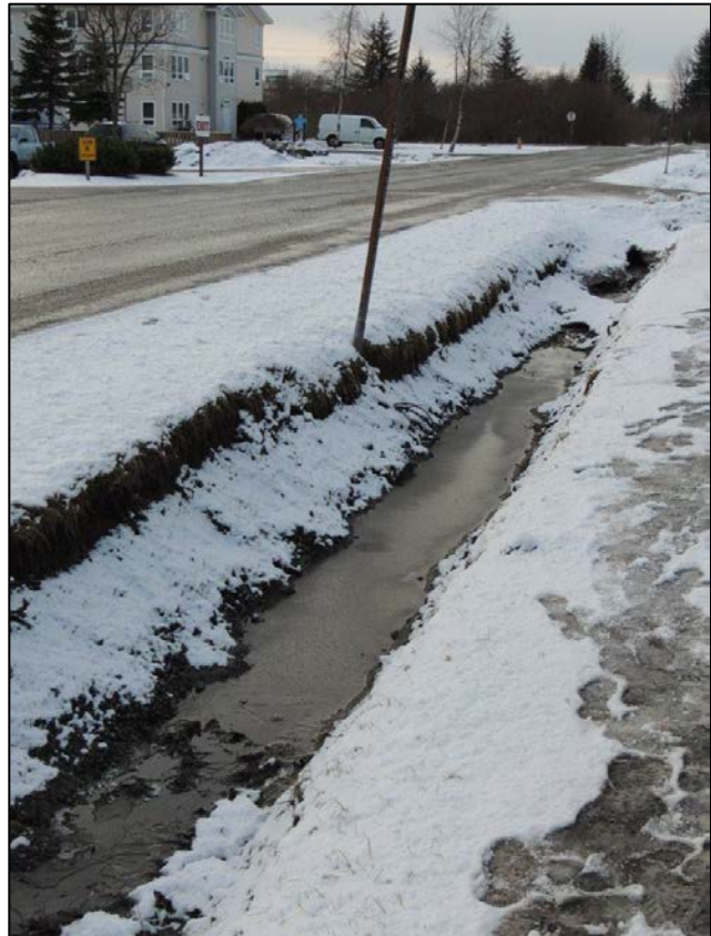
Figure 33. A ditch on the north Side of Teal Street (view looking west from Crest Drive).
