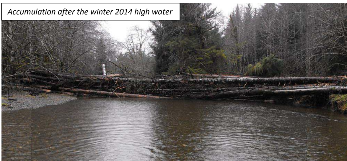
Figure 6. Photos Pre-Post Flood. Looking downstream at the jam downstream of the “hanging pipe” crossing. The large piece of residual wood in the upper photo was originally parallel to the channel on the channel edge prior to restoration. During restoration one end of this piece of wood was moved out into the channel in an effort to deflect flow, induce scour, and create habitat. Early fall flows moved (“spun”) the log to a cross channel location (upper photo) and the January flood resulted in additional wood accumulated on the log. A large, complex, cross channel, log jam has resulted.
