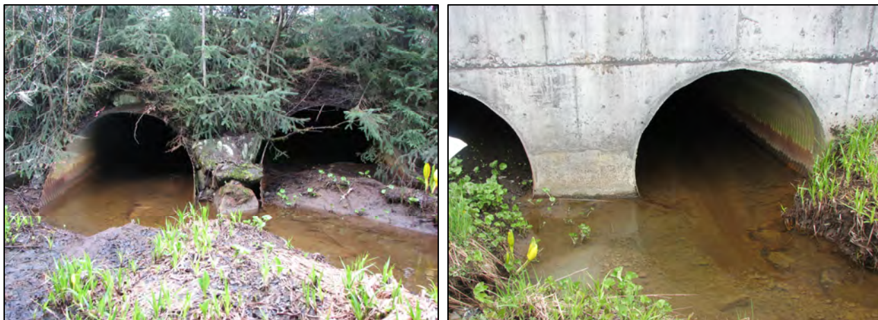
Figure 10. The inlet (left) and outlet (right) of the Glacier Highway culverts. As shown, one of the culverts has failed due to sediment build up.
