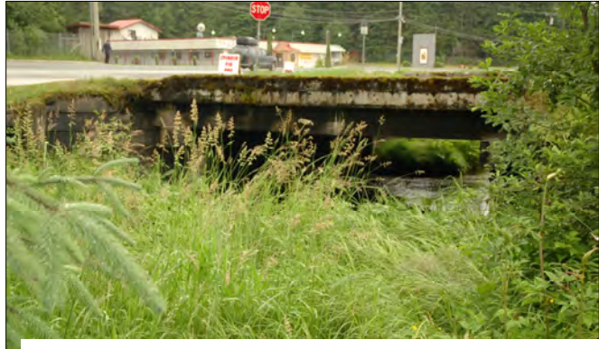
Figure 12. One of the creosote bridges crossing Vanderbilt Creek. Photo by: Eric J. Chandler
