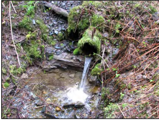
Figure 11. One of several undersized, perched culverts on Vanderbilt Creek along the Lemon Creek Trail
