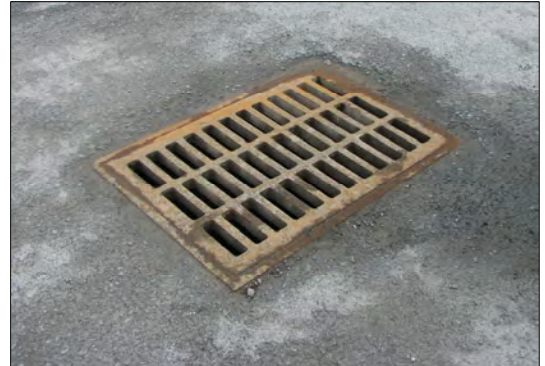
Figure 5. A storm drain on Short Street that transports sediment directly into Vanderbilt Creek.
