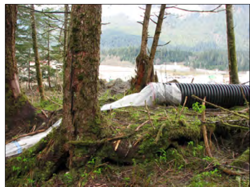
Figure 9. The temporary water diversion conduit that transports stormwater from the hill behind Home Depot into Vanderbilt Creek. June 2007
