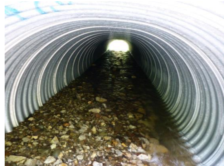
Embedded Structure Tongass N.F.
