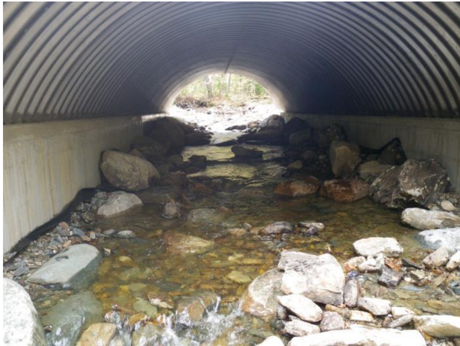
Pre Irene Construction Inside Structure
