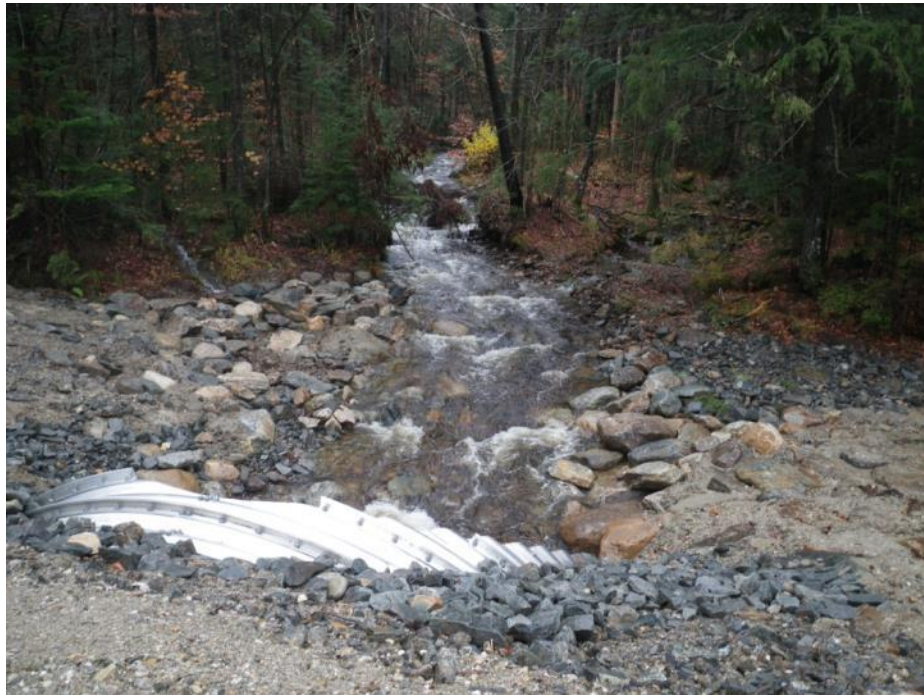
Pre Irene Construction Upstream of Structure
