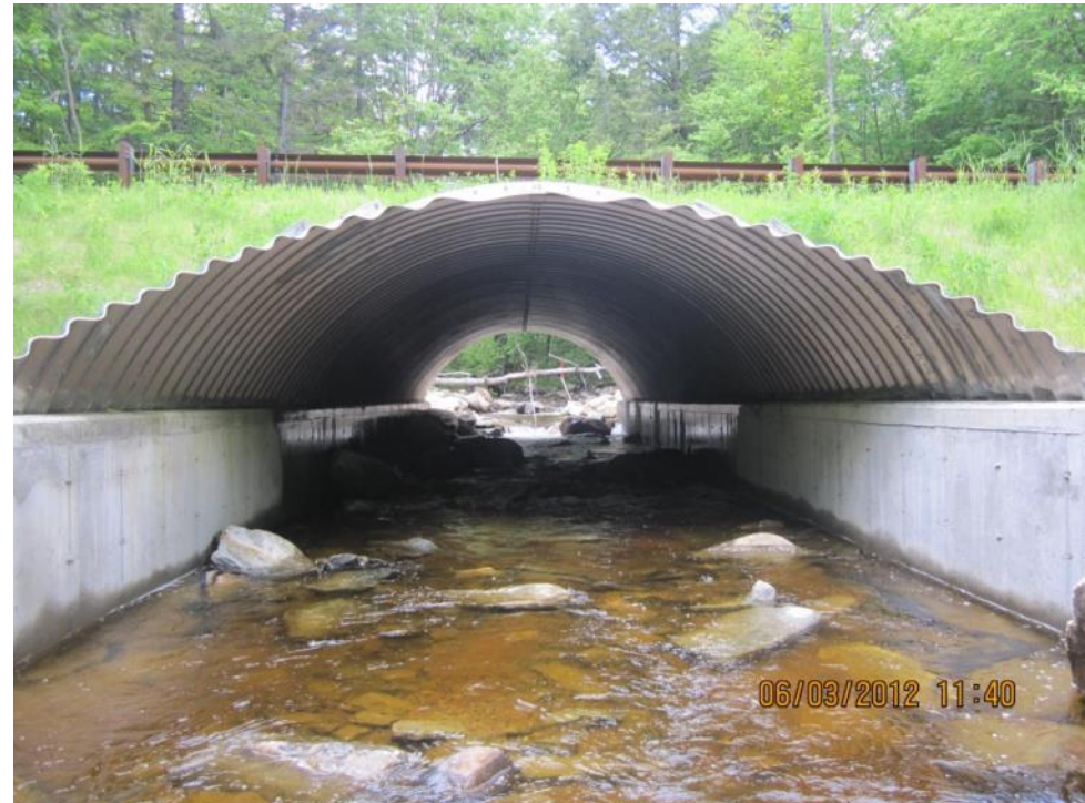
Post Irene Condition Inside Structure
