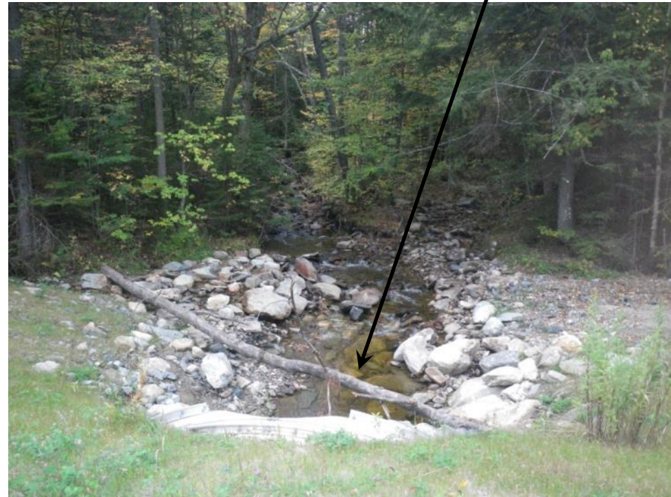
Post Irene Condition Upstream of Structure
