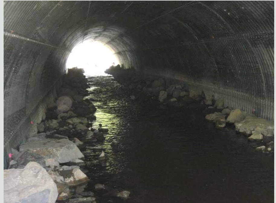
Coal Creek, Kenai (12 foot channel in 18 ft. pipe)
