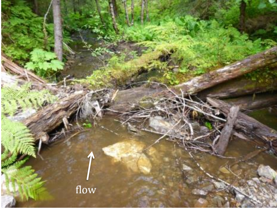
Figure 10. Downstream low stability grade control buttressing upstream sediments within the culvert on 20rd-125.242mp. Loss of this structure would cause a 1 to 2-foot perch at the culvert outlet and remove sediment from inside the structure.
