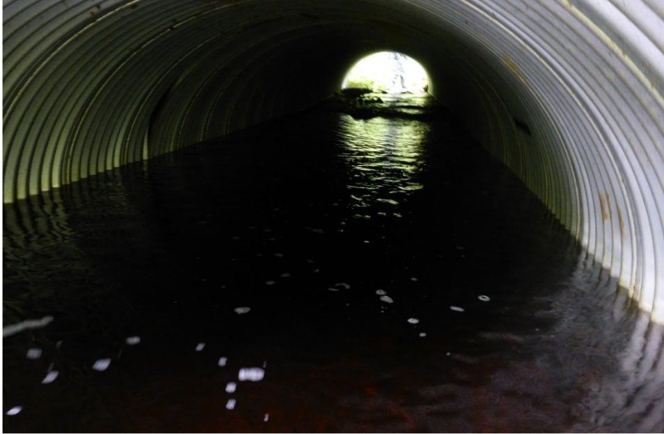
Figure 2. No key pieces present in narrower than bankfull width structure. The wedge of streambed material is at the inlet of the structure, while the remainder of the culvert retained very little of the originally placed stream substrate. Downstream of the outlet the channel may have degraded or the grade control failed.
