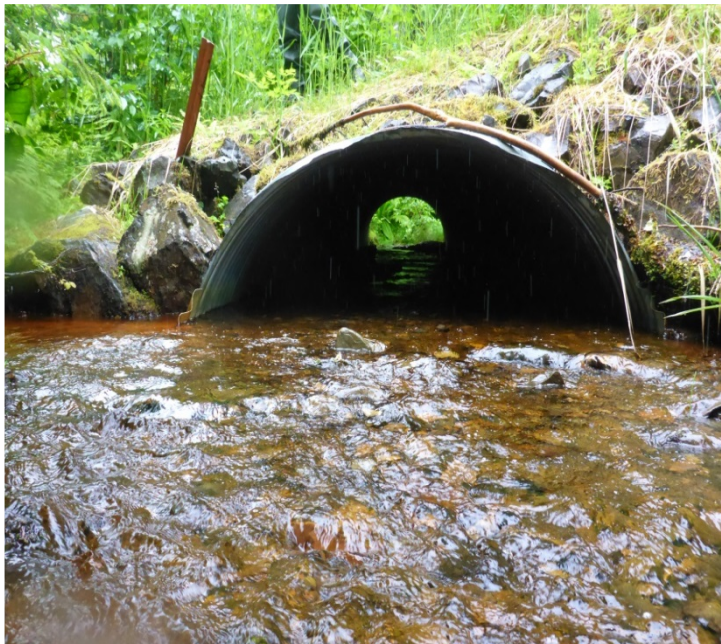
Figure 3. Stream bed aggradation has occurred due to lack of proper inlet and outlet transitions from the culvert to stable stream banks. Leaving over-wide channel from previous undersized structures causes rapid width expansion, which results in sediment deposition. (6415 Road)
