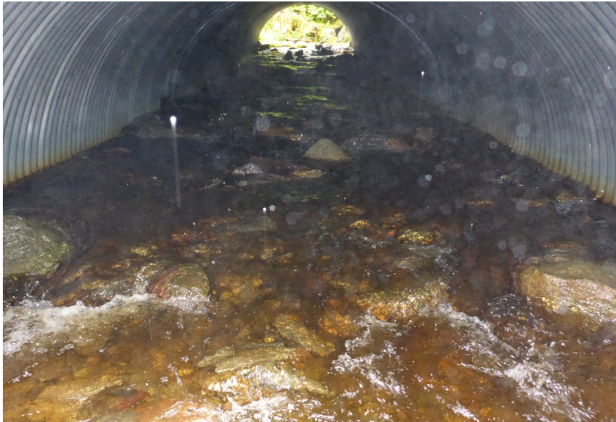
Figure 5 - Bed complexity in 2014, ten years later at same site as Figure 4. (40000 rd - 3.337mp)
