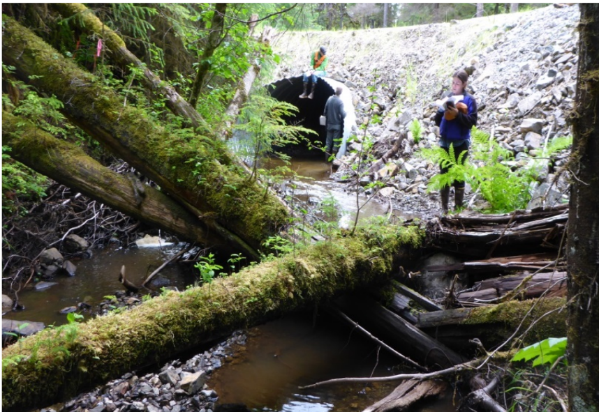
Figure 7 - 20rd-125.242 mp - Natural log grade control immediately downstream of MEAOP design. Logs are in poor structural condition. These rotten and broken logs can easily be lost in future high flows causing loss of substrate within the structure or perching the structure from the tailcrest elevation differential.
