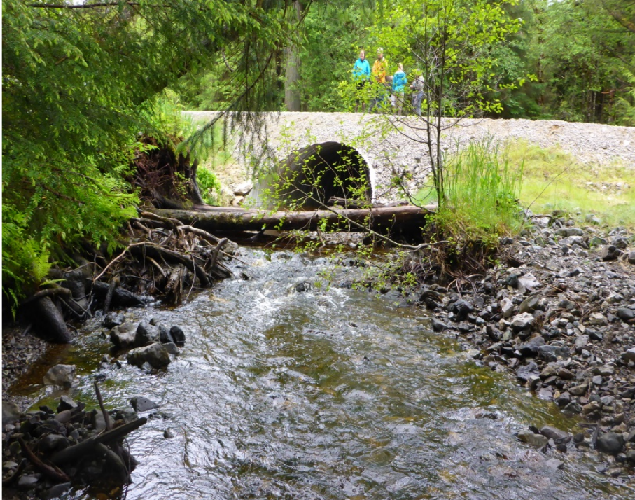
Figure 6 - 20rd-102.907 mp - Note logs in channel immediately downstream of outlet. Wood is excellent habitat for aquatic organisms however its proximity to the outlet pose a risk of future aggradation reducing hydraulic capacity. Shifting the pieces along the margin of the channel would have reduced risk and still provide the habitat component
