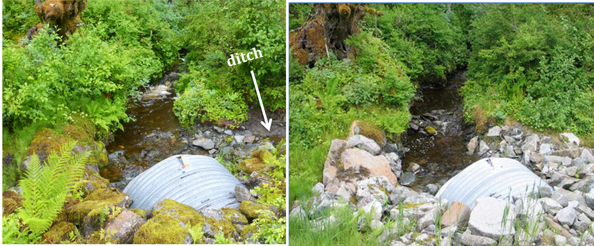
Figure 13. Stream simulation culvert installed in 2002 at 40000rd-2.49mp. Note the removal the bankline on river left from reconstruction of the inboard ditch along the road in the current condition. The culvert is functioning fine, however destruction of bankline could lead to long-term aggradation, reducing culvert hydraulic capacity and decreasing low flow water depths at the inlet.
