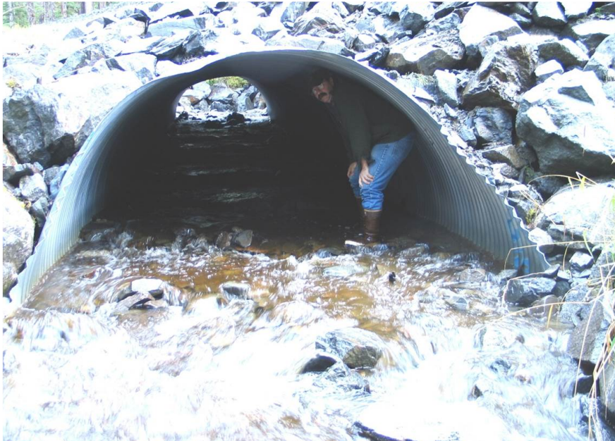
Figure 4. Bed complexity in 2004, similar to that observed in the natural channel. (40000 rd, 3.337mp)
