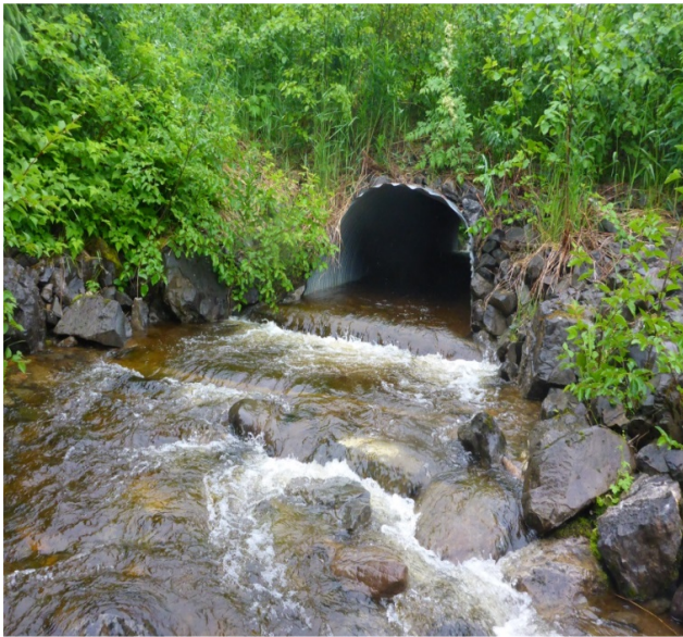
Figure 1. Kuiu Island 6407 road - log and boulder grade controls backwatering the structure and maintaining gravel/cobbles in a structure that is narrower than bankfull width. An additional small cmp was added as a lateral structure to handle flood flows.
