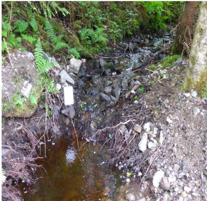
Figure 9. 1.5-foot high headcut moving upstream at 20rd - 0.944mp. Head cut will continue to move upstream until it hits a stable grade control or bedrock.
