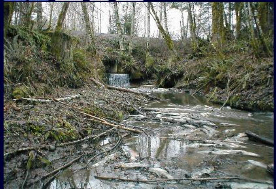
These salmon died because they were blocked by a barrier culvert. Photo from Washington Department of Fish and Wildlife
