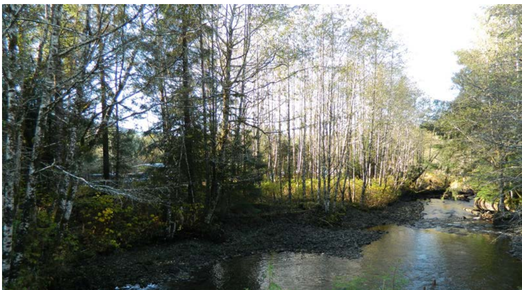
Photo 27. Threemile Creek looking downstream from Klawock-Hollis Highway bridge showing the dike installed by a resident of the Klawock Lake Subdivision, Klawock, Alaska.
